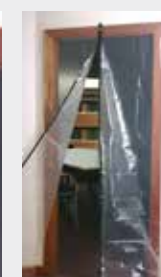
Zip can be opened to allow access and closed to prevent dust spreading
