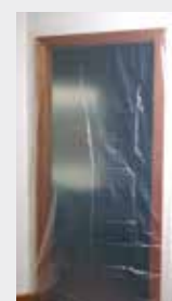
Tape polythene sheet to doorway
